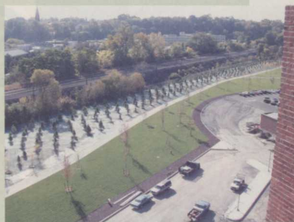
About 700 evergreens were installed between a railroad area and the GE office complex.
