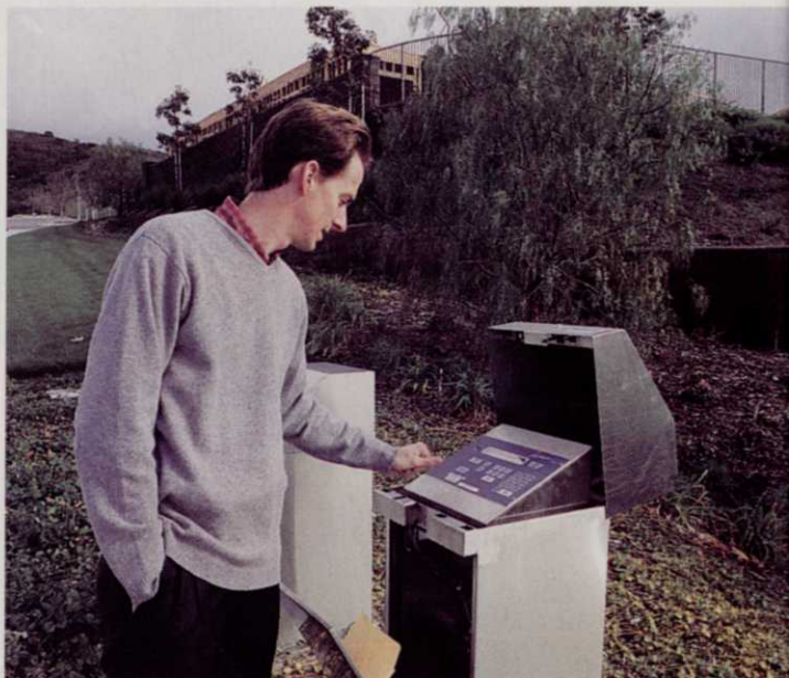
Irrigation consultant Steve Hohl programs one of over 300 Rainmaster Evolution controllers being installed for the Ladera Ranch project.
