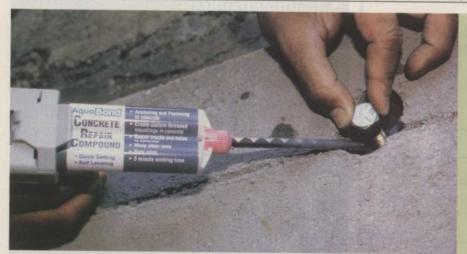
Aquabond's hand-held dispensing and mixing system for its two-component, concrete repair compound dispenses compound for custom threaded mounting and fastening. The compound is dispensed around a lubed bolt and then allowed to dry. The bolt is then unscrewed, creating a custom thread for easy removal. For more information contact Aquabond at 714/685-4922 or circle no. 281
