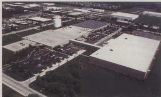
Echo Incorporated, Inc., Lake Zurich, IL facility
