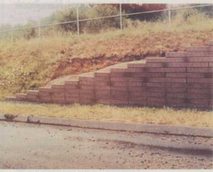
▲ Barco Products' recycled plastic landscape timbers are perfect for small retaining walls, walkway and garden edgings, planters and pond enclosures. They resist rotting, splintering and insect damage. The timbers measure 8 ft. X 5.5 in. X 5.5 in., feature an interlocking edge and pre-molded knockout holes for rebar rod reinforcement, and can be cut and drilled with conventional hand tools. For more information call 800/338-2697 / circle no. 277
