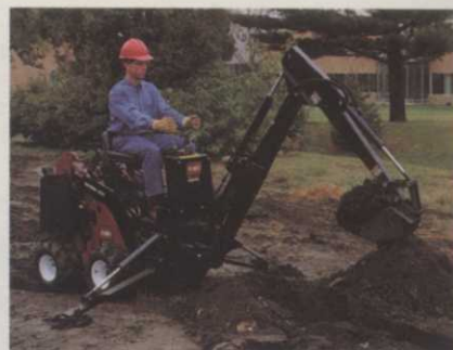
Toro SiteWork Systems with backhoe
