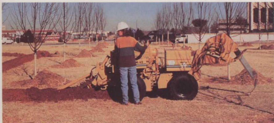
Davis Landscaping, Harrisburg, PA, uses a LM-42 to plow in the laterals.
