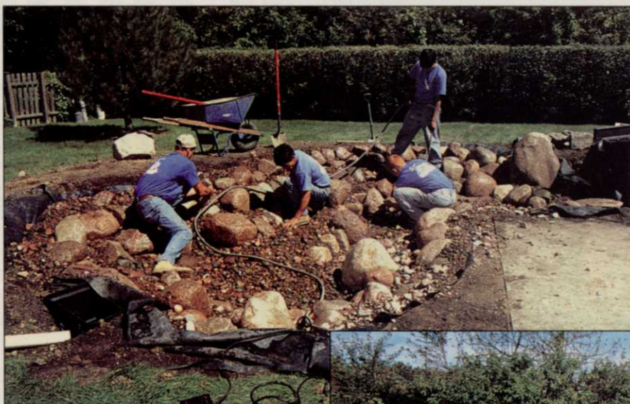
Left: wash off the rocks by using a garden hose while washing the dirt into the sump pump at the bottom of the pond. Bottom: Two or three tons of cobblestones are used around the berm for support. (Photos courtesy Aquascape Designs)
