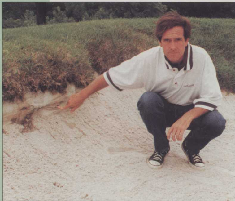
Kelch shows the filter fabric liner at hole 17 that has become exposed due to raking. It's tough to keep the grass wet and growing over the liner, says Kelch. The liners will be removed before the Bell Atlantic tourney.
