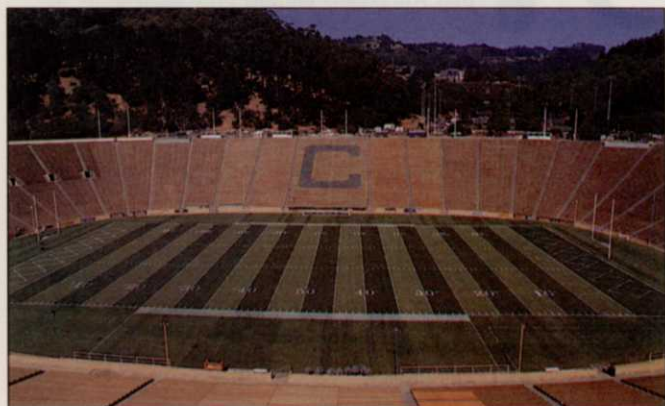
CMX Group designed, oversaw the 5-month Memorial Stadium construction project and installation of new Kentucky bluegrass field.
