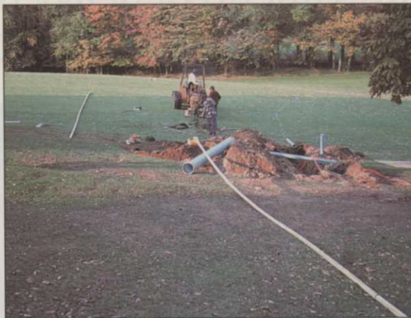
Lateral pipe and wire are installed with vibratory plow.
