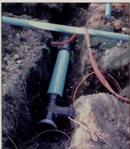
Main line tees are ready for thrust blocking.
