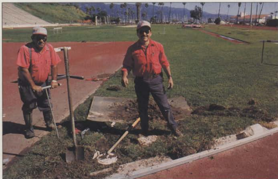
Crew chief Nacho Garcia, left, and Ricardo Valenzuela do such good work that most irrigation installations at SBCC are done in-house. A 12-person crew keeps the college green.
