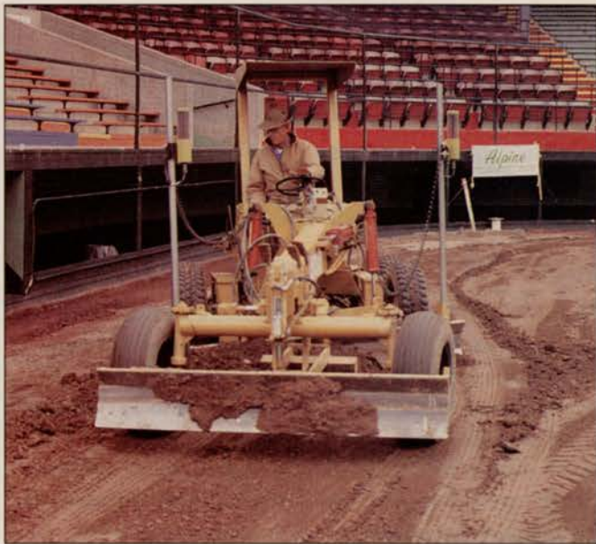
Grove Teates of Alpine Services used a laser to make sure Little League's World Series field drained to the warning track, foul lines.
