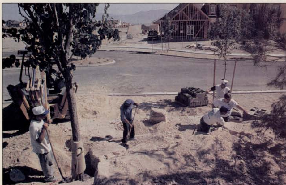
A Par-3 Landscape residential construction site in the Mountain Trails subdivision—workers installing mature trees to give a finished look to an upscale job
