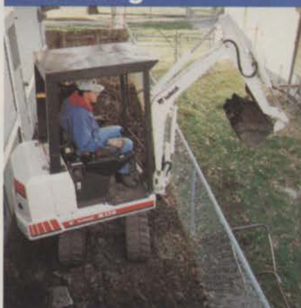
Replacing Drain Tile
