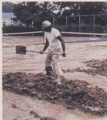
Soil erosion ruined this tennis court.
