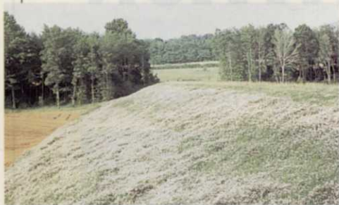
A thick turf cover protects underlying soil on slopes.
