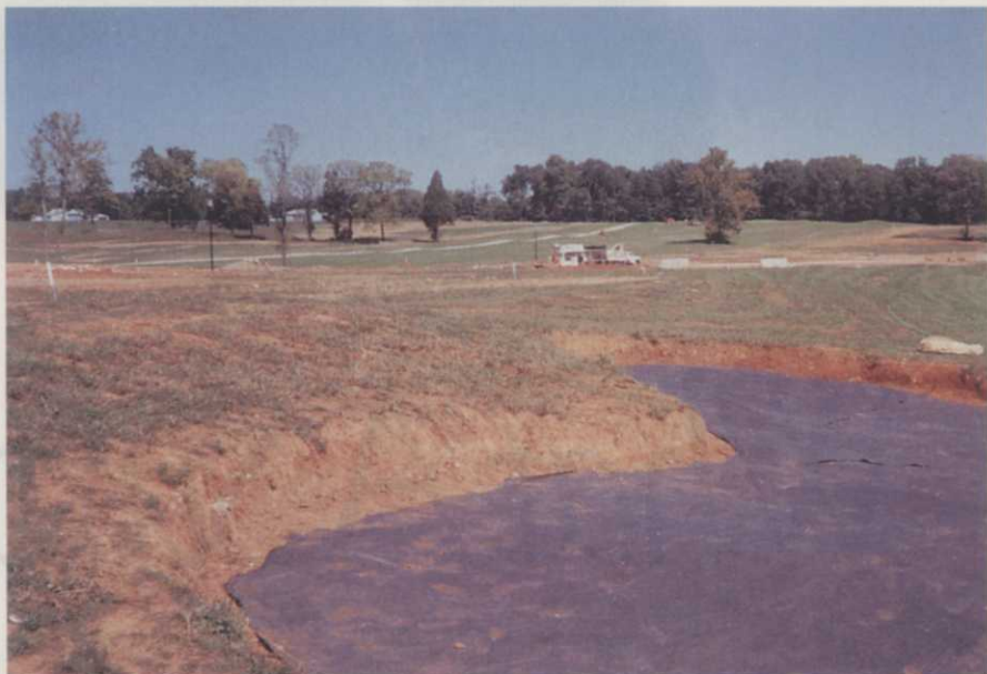
Phillips Fibers' Supac geotextile fabric separates sand from subsoil in bunkers, helps filtration and drainage, and provides structural stability.
