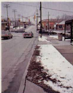
Primary salt damage is found along areas along roads.
