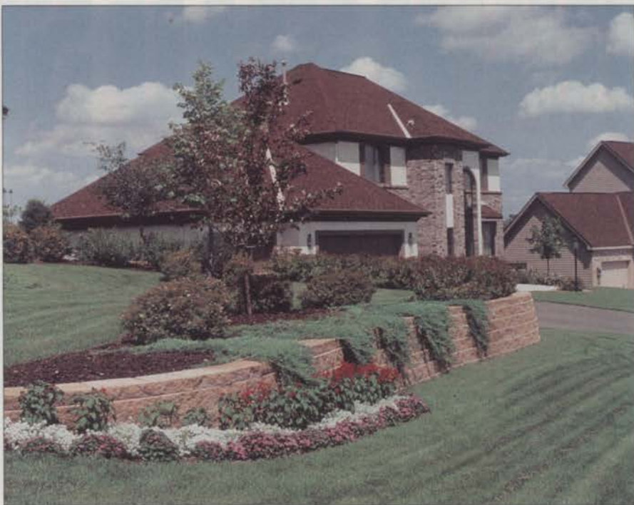
Stone-faced block wall helps set off a stunning residential landscape.
