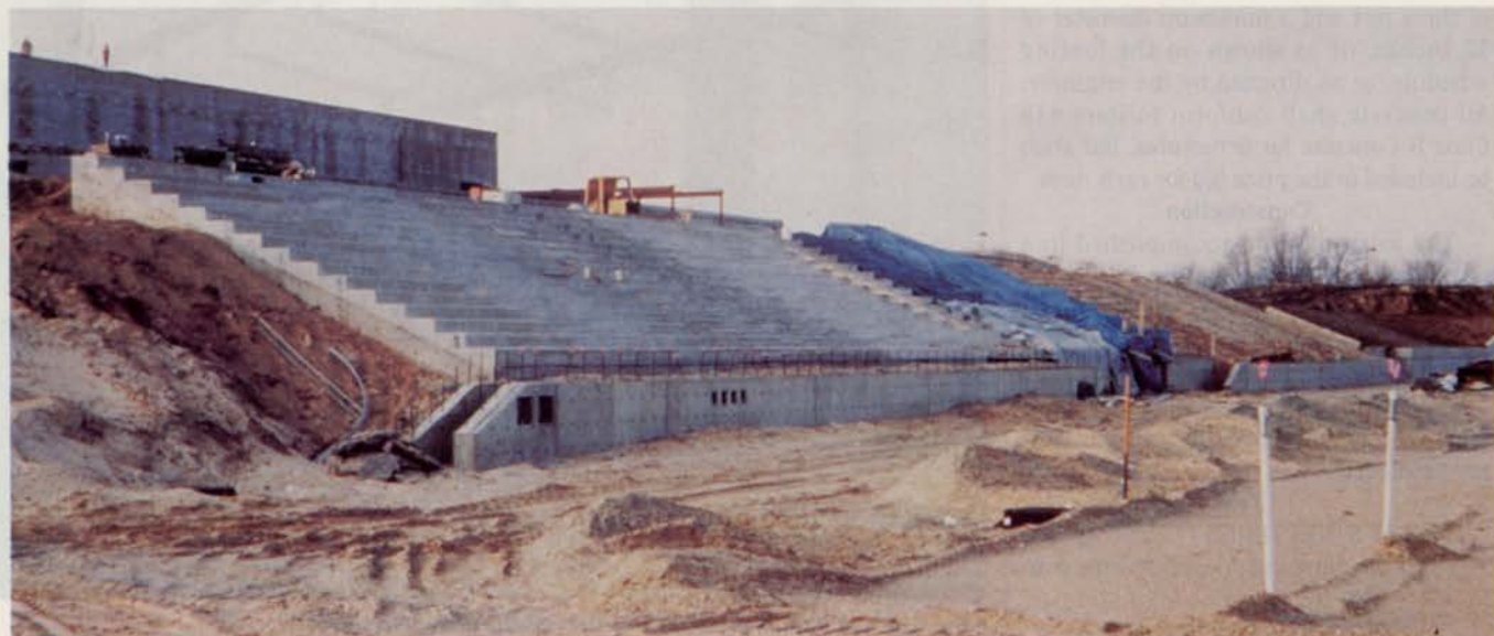
New Rockford High Stadium being built into slope for beauty, cost savings.
