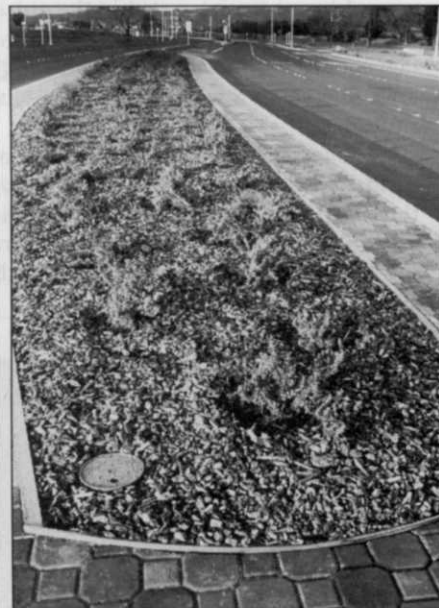
TechLine makes it possible to irrigate curved, angular, narrow median strips without overspray and water run-off.
