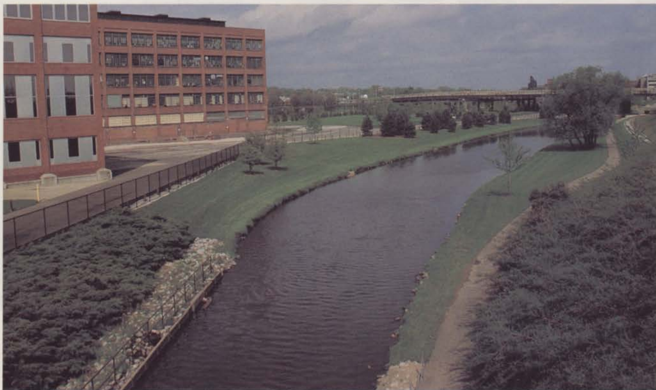
Green space along the Ohio Canal is fully maintained by Goodyear maintenance crews. The canal is one of three sources of water for irrigation and plant operations.
