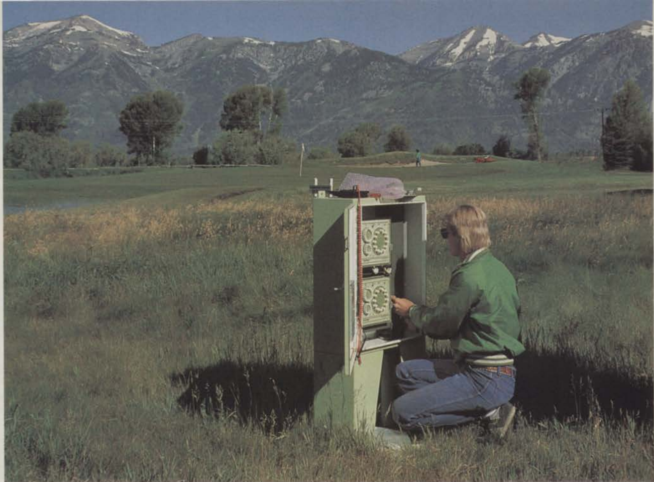
Superintendent Brian Heywood opens his gear drive and impact rotors before using a 185 or 205 cfm air compressor to blow out all the water.
