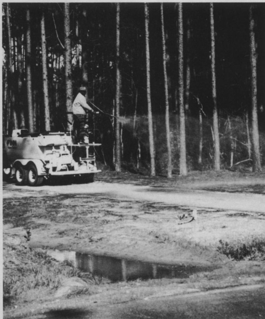
In addition to the playing surface, many areas—such as cart paths—require continuous management to maintain the desired condition. Using a tower gun or remote hose method of hydro-seeding makes it easy.
