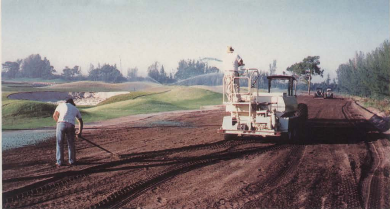
The Polo Trace Course in Florida involved 70 to 75 acres of hydroseeding. Bahiagrass and perennial ryegrasses were used in the roughs and bentgrass on the greens.
