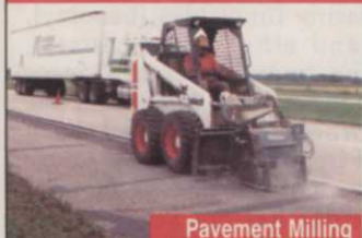
Pavement Milling
