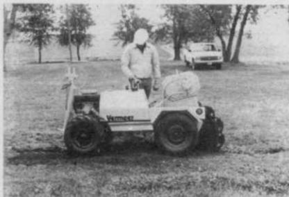
"Sticher" is simple to operate and easily outperforms ineffective hand tampers or make-shift methods that use expensive backhoes to "mash" soil.
