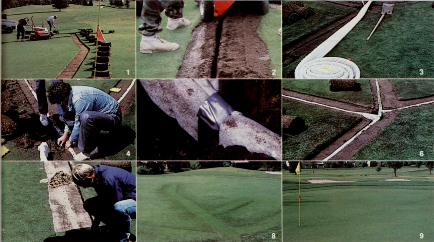
1. Rolling back sod where TerraFlow lines will run. 2. Cutting 2" wide trench. 3. Laying TerraFlow lines in 12" deep trench. 4, 5. Joining TerraFlow lines using only a utility knife and duct tape. 6. Fully installed TerraFlow System. Workers backfill with site soil, puddle with sand. 7. Replacing sod. 8. Completed TerraFlow System. Installation time: about 100 ft. per hour. 9. Green was back in play in 2 hours with TerraFlow. (Photos by Greg Fast, Turf Irrigation Supply, Englewood, Colorado.)
