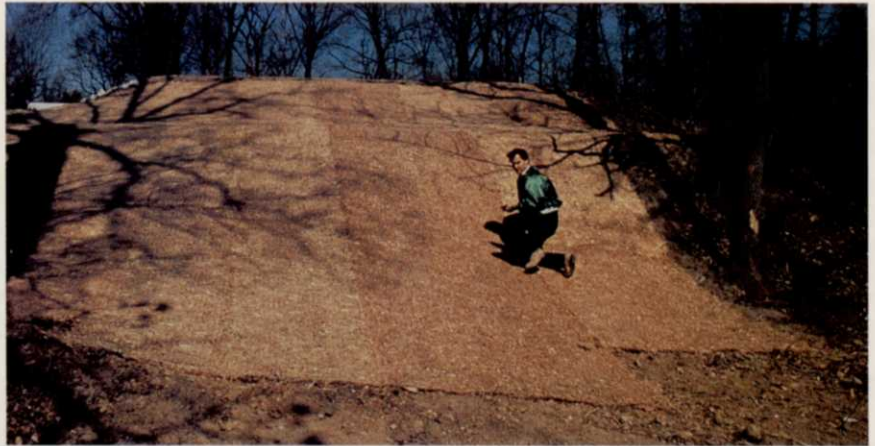
After seeding, erosion control blankets are installed.
