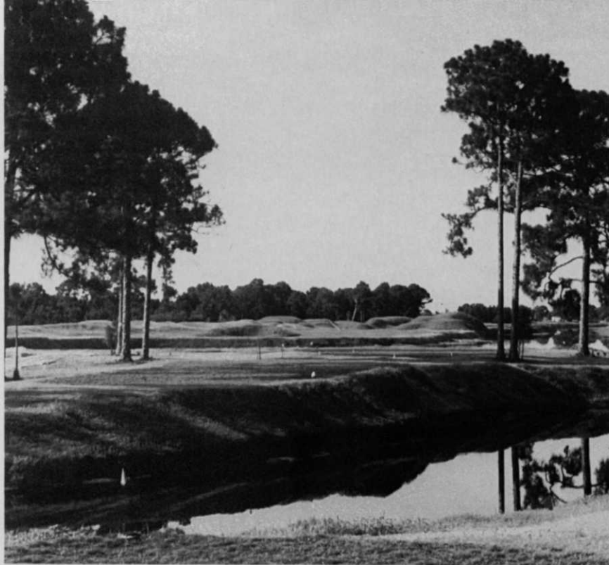
Shown here is hole No. 5 while under construction. That hole has been made even more difficult by a man-made marsh surrounding it.
