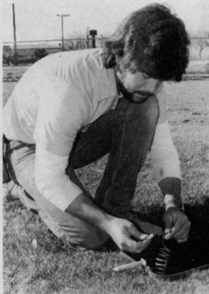
Connecting the second of 3M DBY Direct Bury Splices is equipment operator Christopher M. Cabral. The self-contained DBY kit, with nothing to lose and no sealant tubes to dry out, is invaluable to Warner's because its jobs are often in remote areas.
