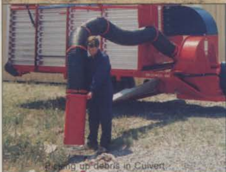
Picking up debris in Culvert
