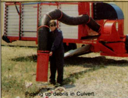
Picking up debris in Culvert.
