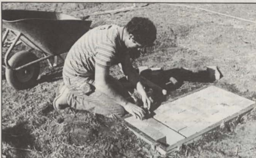
A candidate sets bricks in a running bond pattern according to specifications in the brick-on-sand portion of the CLCA's certification test. The exam took place last October at Football College, Los Altos.
