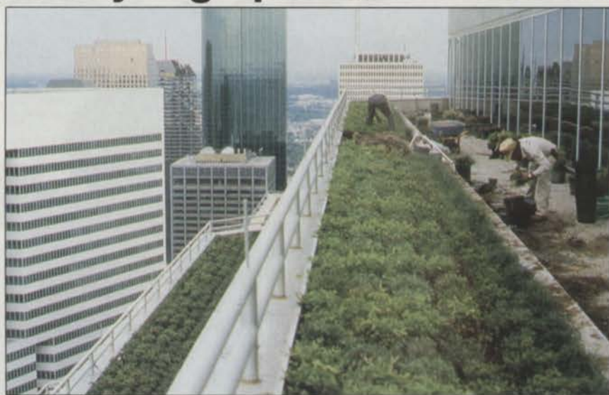
Plants are positioned near natural wind-breaks at the Gulf Tower Building.
