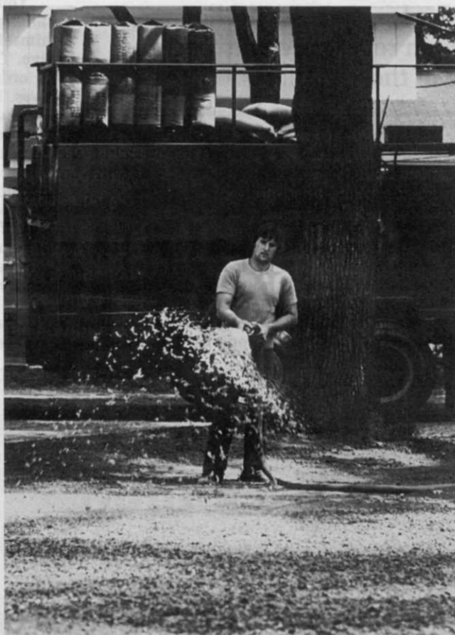
Hydraulic mulching helps establish a uniform stand of turf.
