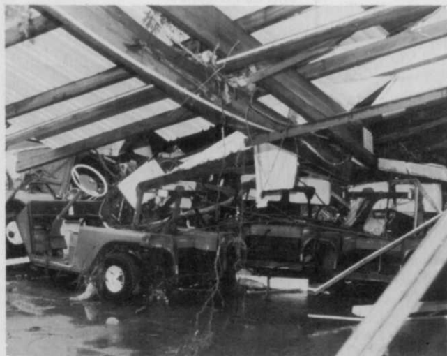
A shed crumbled under the raging current, damaging some golf cars.
