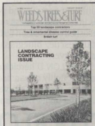
The Prudential's Freedom Business Center in Valley Forge, PA.
