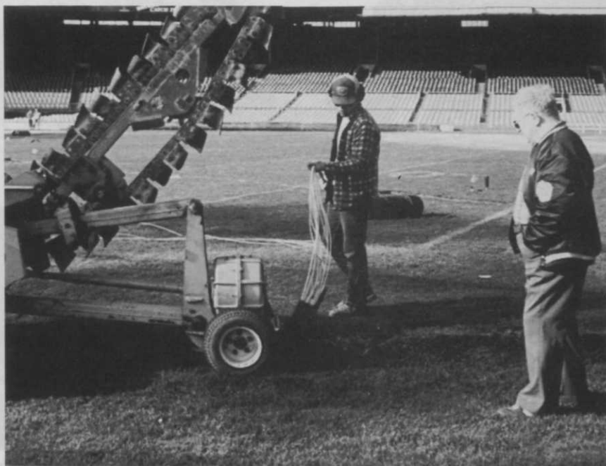
Harry Gill (right) supervises installation of the irrigation pipe and wires through slit sod. "The only places we had to remove the sod was when we came to a sprinkler head," Gill notes.
