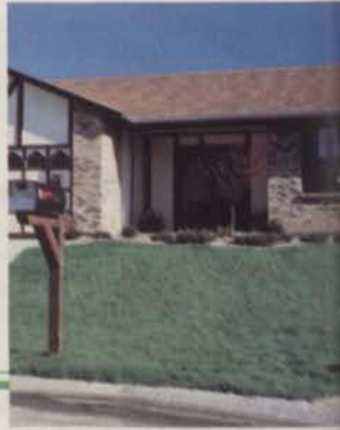
5. COMPLETED RENOVATION DAY 30
