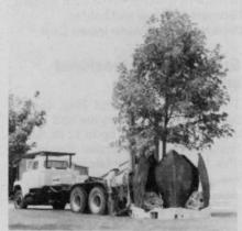
mize limb clearance inside the spade, and a maximum rear-half height of 85 in. allows operation close to other trees and structures. A dual control system allowing operation from cab or next to rear-half assembly is optional.
