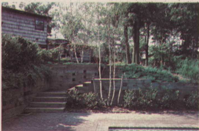
Dubner — Steep lot presented challenges of a pool and low maintenance material.
