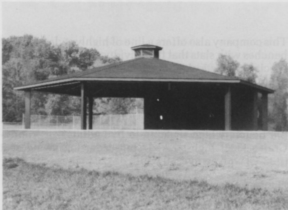
A hexagonal park shelter by W. H. Porter may be partially enclosed for rest rooms and storage.
