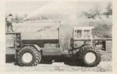
chassis, the hydro-mulcher can traverse remote areas where large trucks can't reach and where truck tires might harm existing ground cover. The four-wheel drive Ag-
