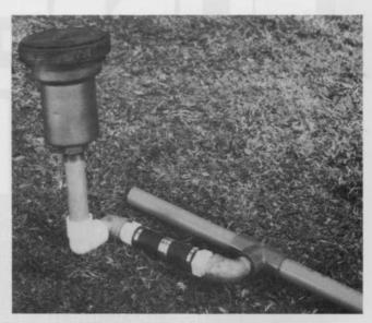
Extra steps during installation save in repair time later, such as this device which protects both heads and pipe from damage.
