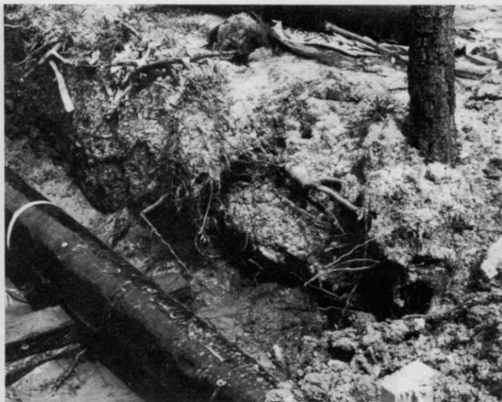
Underground utilities often cut many tree roots and cause a decline in nearby trees.
