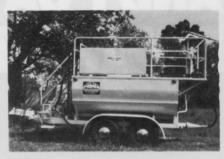
The Ero-Con Machine is the latest design concept in equipment from Strong Manufacturing Company. It is designed to gently mix and sprayapply all varieties of mulch (wood fiber and cellulose), seeds, fertilizers and lime.
