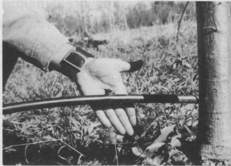
Emitter , inserted directly into laterals through a hole punched at the base of each tree, simplifies and shortens the installation process.
