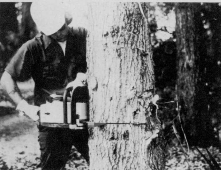
Wedge behind saw in cut prevents chain binding (left). Protective clothing (right) includes gloves, hard hat, and eye and ear protection.
