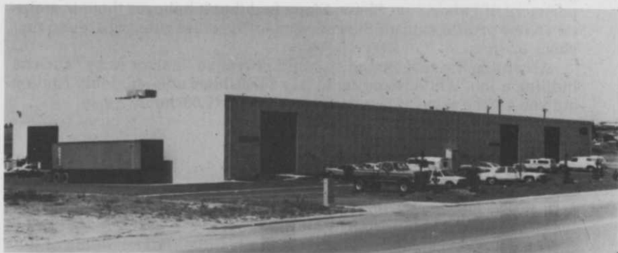
Ferrari International, Inc. has completed its move to new corporate headquarters in San Marcos, California. President Harold Sankey said, "Our sales have doubled in the last three years and this new building will form the basis for our projected growth."
