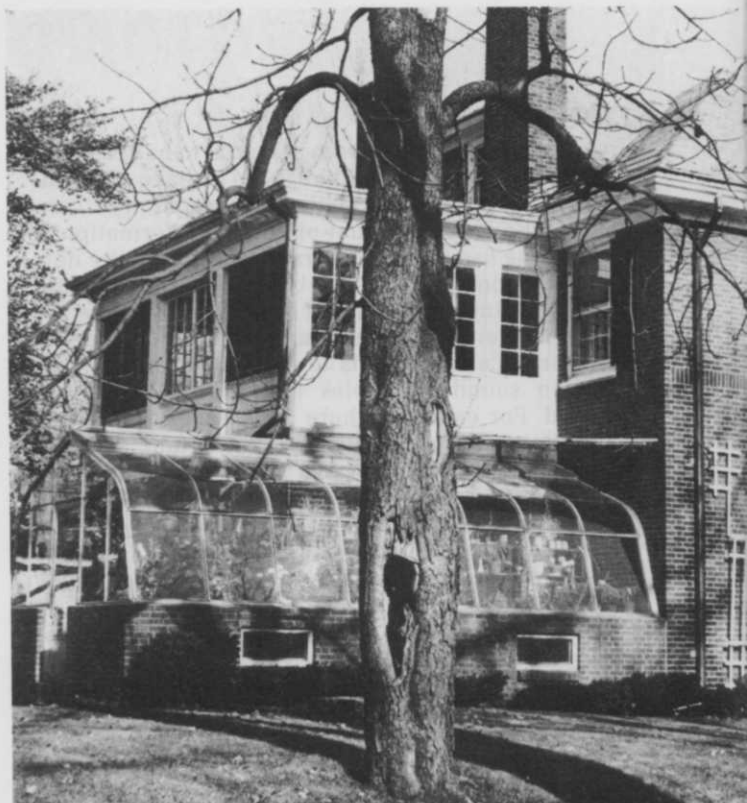
A decayed tree posing a threat to a greenhouse and residence. Too often people learn about decay too late.
